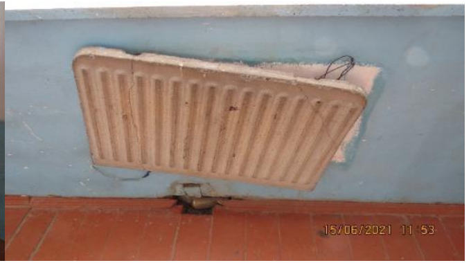
Description: Building after retrofitting
