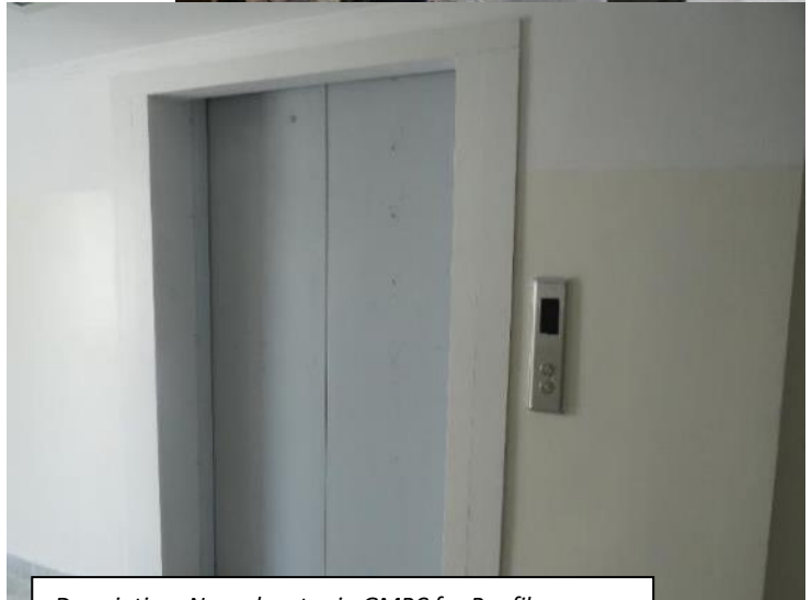
Description: New elevator in GMPC for Panfilov rayon
