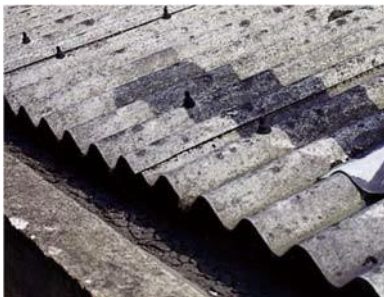
AC sheets used as roofing
